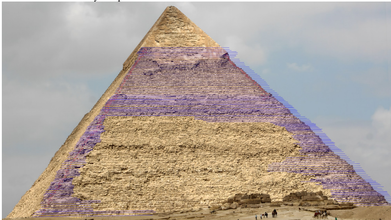
Fig. S6.1. Semi-automatic extraction of masonry-course profiles from a frontal image of the Pyramid of Khafre. Horizontal guide lines (blue) were manually aligned with visually identifiable masonry courses across the pyramid face and subsequently processed using a custom line-detection workflow developed by the author. The software identifies line centroids, merges adjacent detections within a configurable threshold, and converts vertical pixel spacing into approximate real course heights using the known visible height of the pyramid as a scaling reference. The method is intended to detect relative variations in course thickness, discontinuities, and large-scale geometric patterns rather than to provide absolute architectural metrology. Photo by Carlota O. on Unsplash, used under the Unsplash license (accessed January 31, 2026), blue lines created by the author.
