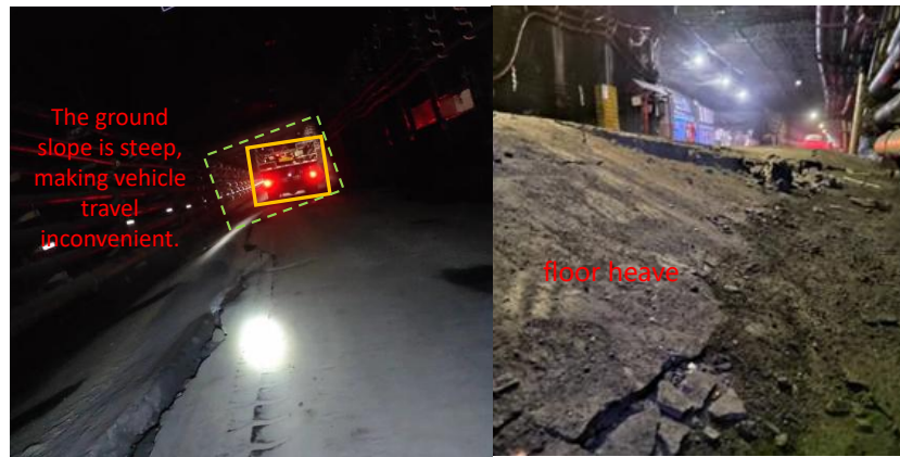
Fig.2 Roadway deformation
