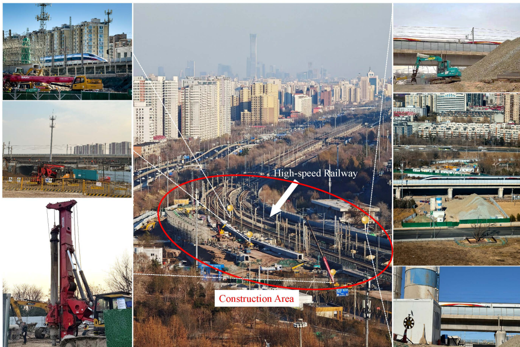
Supplementary Figure 5 | Panoramic and close-up photographs of the construction site.
