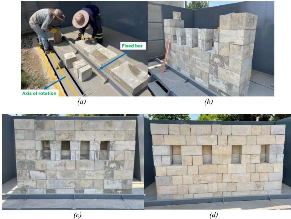
Fig. 9 Construction of the walls: (a) Placing the first course, (b) Arranging the upper blocks, (c) Wall A-1 completed (model A), and (d) Wall B-1 completed (model B)
