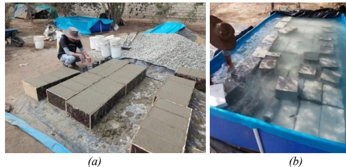
Fig. 7 Concrete blocks: (a) Making blocks, and (b) Curing of concrete
