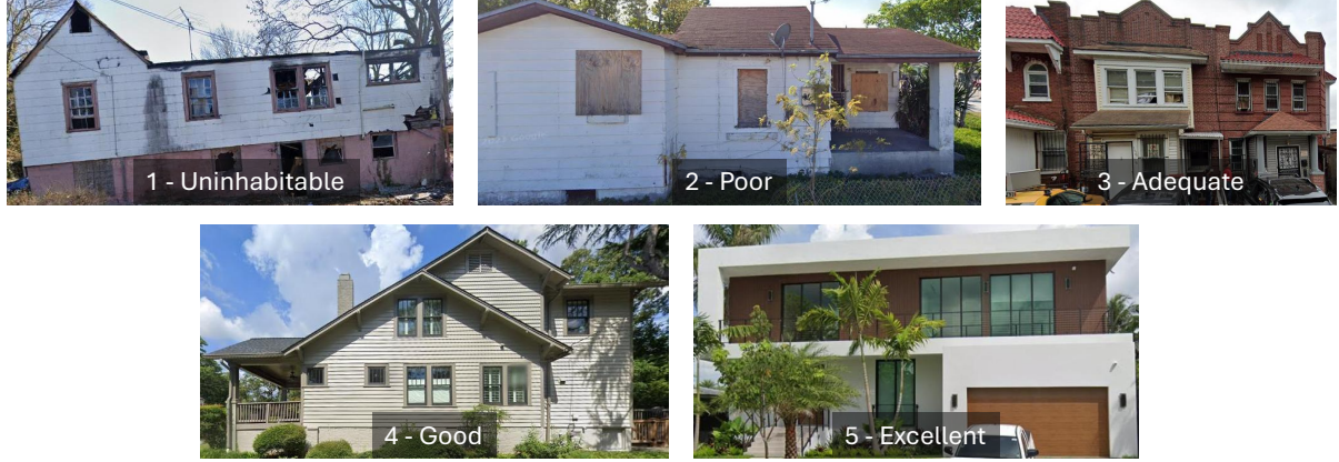
Fig. 2: Examples of buildings corresponding to each condition rating.
