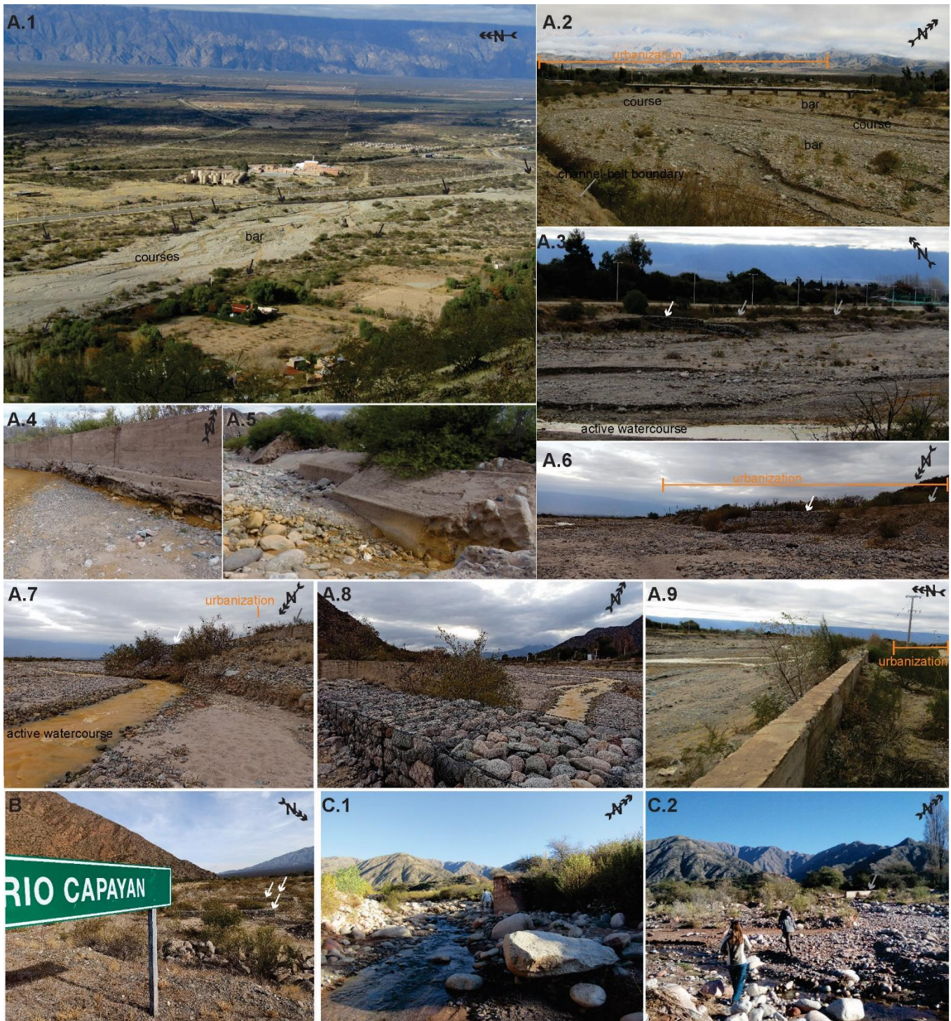
Fig. S7. Retaining structures associated with fluvial channels. A) Channelized segment of the Los Sarmientos River and adjacent urbanized areas. A.1) Braided channels, bars, and retaining structures (black arrow). View from the Sierra de Paimán ( 29^{\circ}09'17''\text{S} / 67^{\circ}29'19''\text{W} ). A.2) Braided channels and coarse sediment bars. Active and inactive channels ( 29^{\circ}09'09''\text{S} / 67^{\circ}29'15''\text{W} ). Urbanized area shown in orange. A.3) Retaining structures along the left bank of the Los Sarmientos River: concrete wall (gray arrow) and gabion structures (white arrow). A.4) Detail of retaining structure on the left riverbank ( 29^{\circ}09'28''\text{S} / 67^{\circ}28'26''\text{W} ) showing basal degradation. A.5) Structure on the left bank affected by fluvial action ( 29^{\circ}09'21''\text{S} / 67^{\circ}28'40''\text{W} ). A.6–A.7) Retaining structures on the right bank of the Los Sarmientos River: rigid wall (gray arrow) and gabions (white arrow). Urbanized area in the background ( 29^{\circ}09'12''\text{S} / 67^{\circ}29'06''\text{W} ). A.8) Close-up of the structures shown in A.7 and their interaction with the active channel ( 29^{\circ}09'16''\text{S} / 67^{\circ}28'59''\text{W} ). A.9) Detail of rigid wall ( 29^{\circ}09'12''\text{S} / 67^{\circ}29'10''\text{W} ). B) Capayan River – gabion structures. C) Miranda River: 1) 29^{\circ}20'09''\text{S} / 67^{\circ}39'24''\text{W} ; 2) 29^{\circ}20'09''\text{S} / 67^{\circ}39'22''\text{W} .
