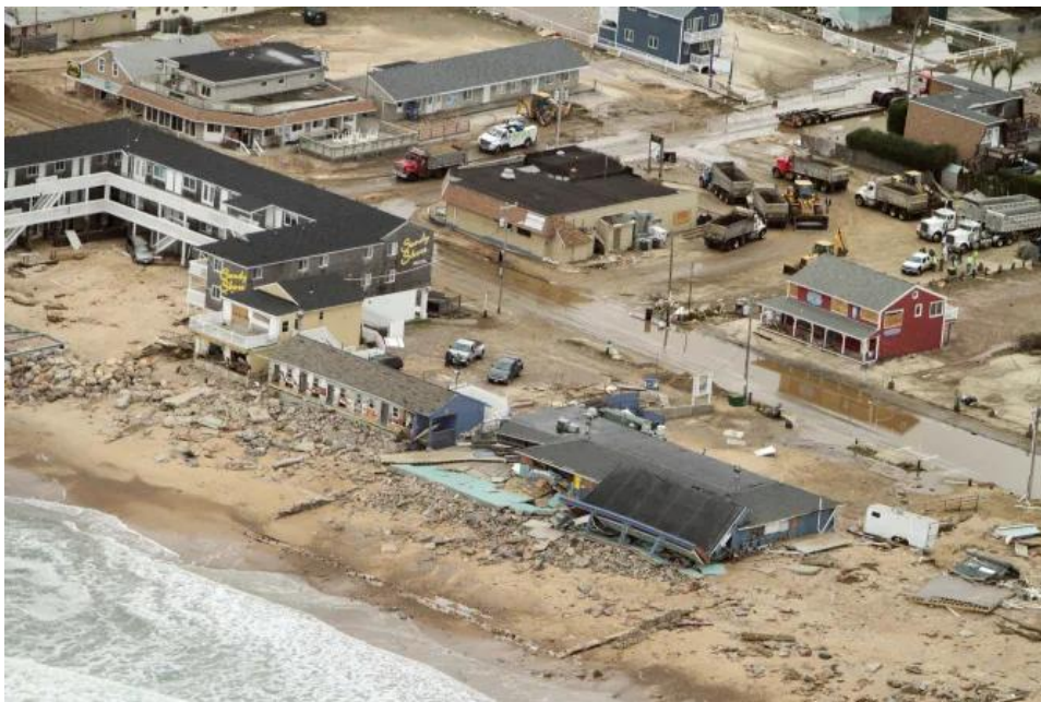
Fig. 3 Damage to Rhode Island’s southern coast caused by Hurricane Sandy, 2012 (Figure: The Providence Journal)
