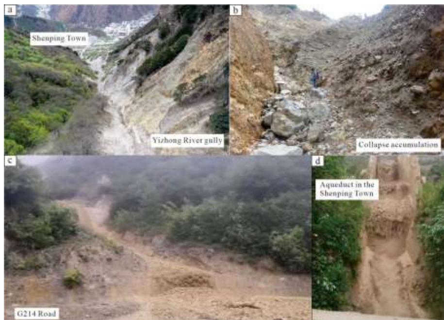
Fig. 2 (a): Overview from the Yizhong River gully to Shenping Town; (b): Large amount of rockfall accumulation within the channel; (c): Impact of the debris flow outbreak on the G214 Road; (d): Scouring of a culvert in Shenping Town caused by the debris flow.
