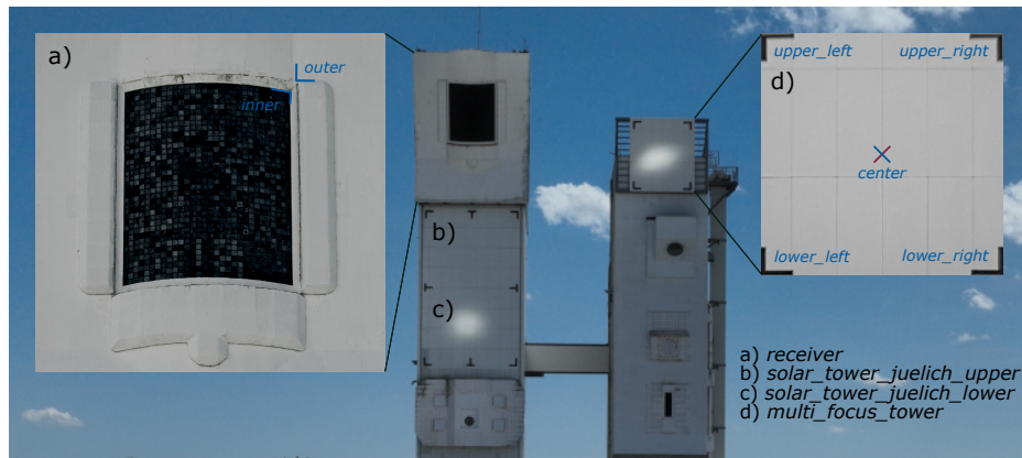
Fig. 1: The tower coordinates. An overview of the coordinates provided in the tower properties data. For the calibration targets only the outer borders and the center are provided, whilst for the receiver both inner and outer coordinates are supplied.
