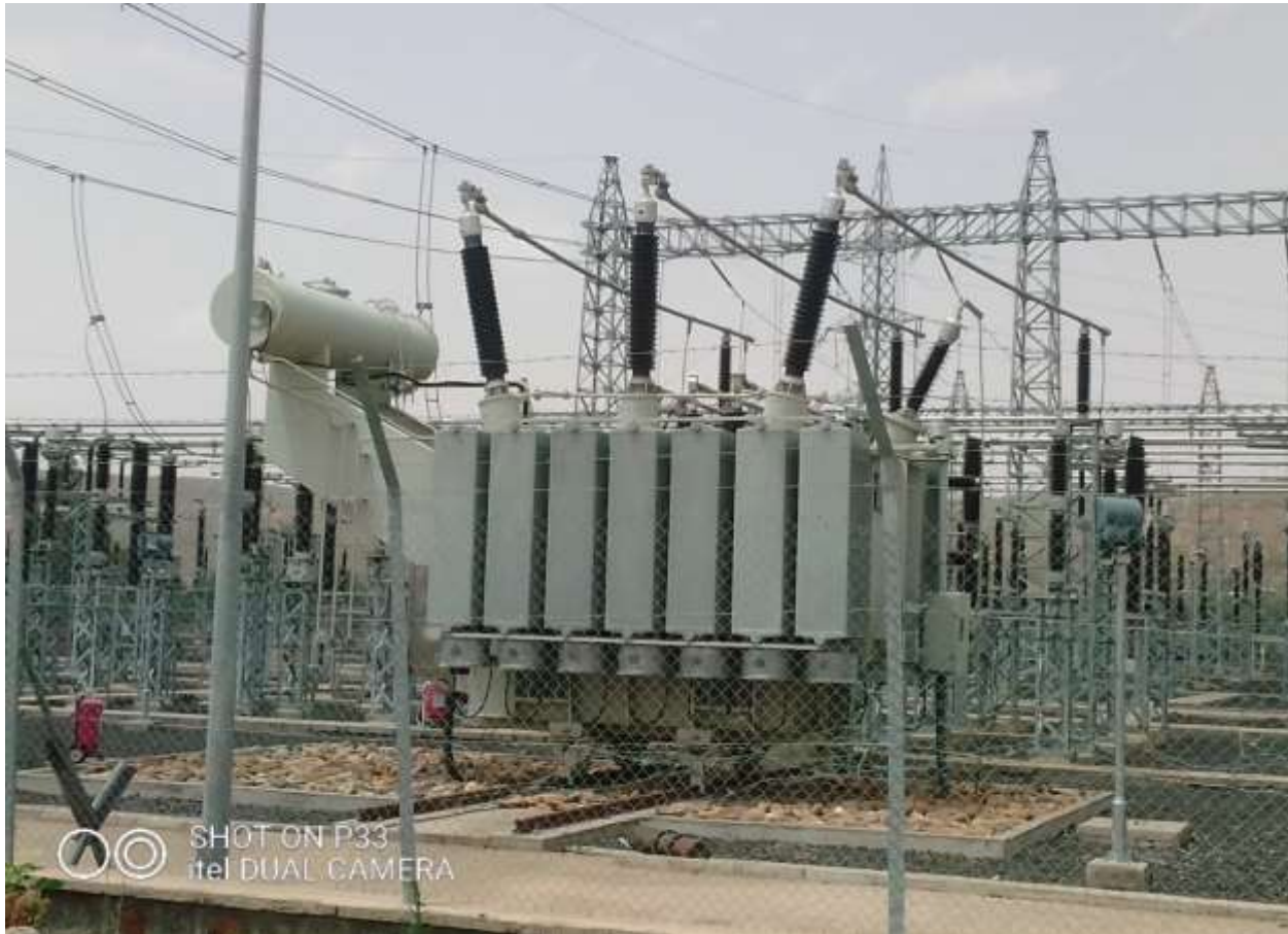
Fig. 1.4: Aksum substation topographic view [3]
