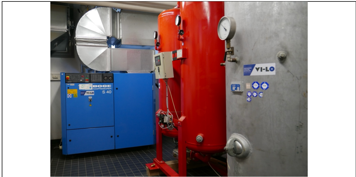
Figure S1 The main parts of the system generating a continuous supply of CO 2 -free air. From left to right: air compressor (blue), self-regenerating adsorption dryer (red), and air receiver (grey). For technical detail, see main text.
