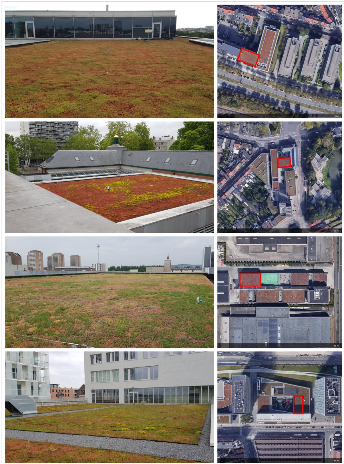
Fig. S3 The investigated extensive green roofs in Antwerp (left), and its Google Earth locations (right). From top to bottom: R9 (conventional; July 2019), R10 (conventional; June 2019), R11 (biodiverse; June 2019), R12 (biodiverse; June 2019).
