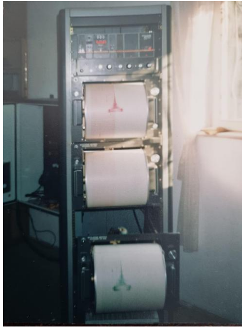
Figure 22. Teledyne Geotech S13 seismometer (recording system) installed at Buzias seismic station in 1983
