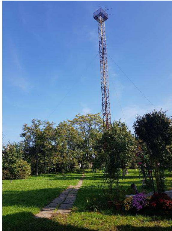
Figure 24. The radio tower was installed in 1995 at the Timisoara Seismological Observatory for radiolink data transmissions from the BZS, BANR, and SIRR seismic stations.
