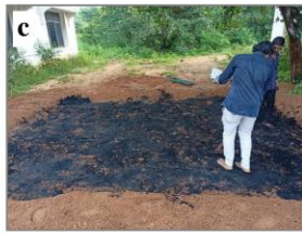
Spreading of stabilisers
