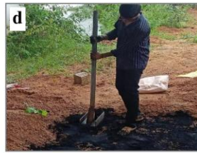
Compaction of the layer
