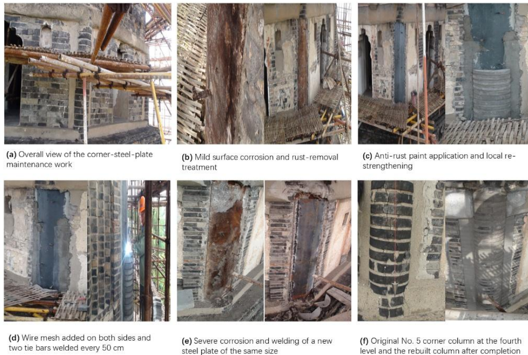
394 Fig. 5. Representative procedures for the treatment of corroded corner steel plates at the Yunyan 395 Temple Pagoda
