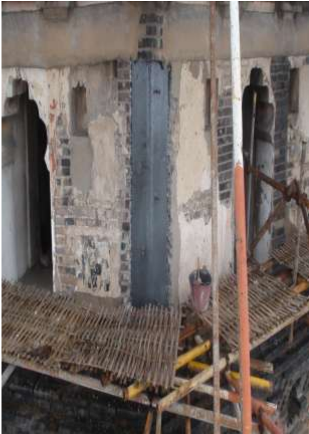
Application of two coats of anti-corrosion coating after rust removal
