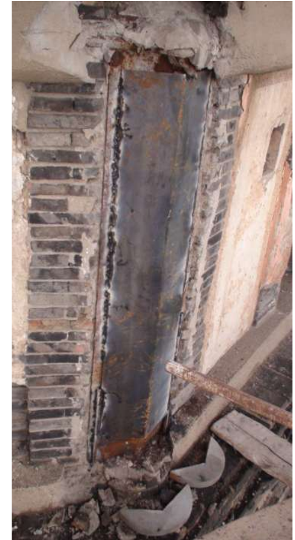
A new steel plate of matching dimensions welded to the retained original plate
