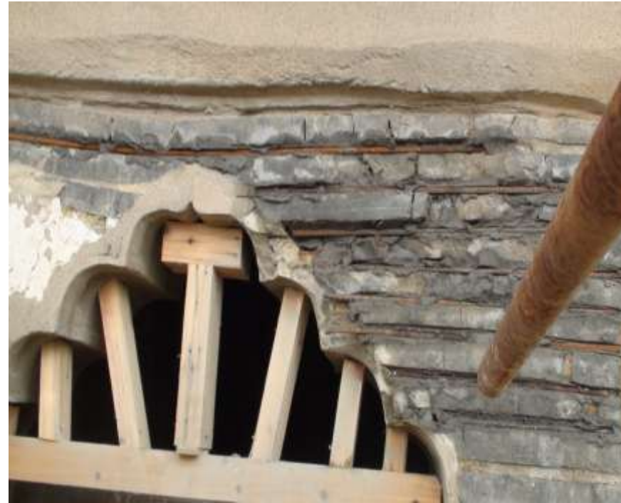
Reinforcing bars inserted into each groove
