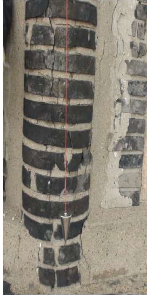
Original condition of corner masonry column No. 5 at the fourth level
