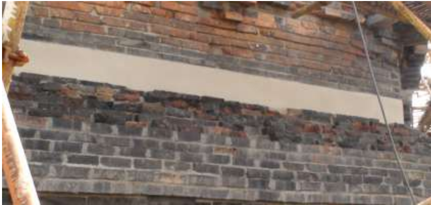
After local repair
