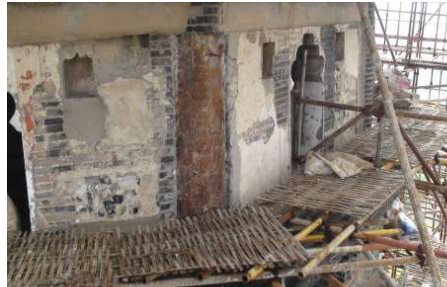
Removal of loose surface corrosion products
