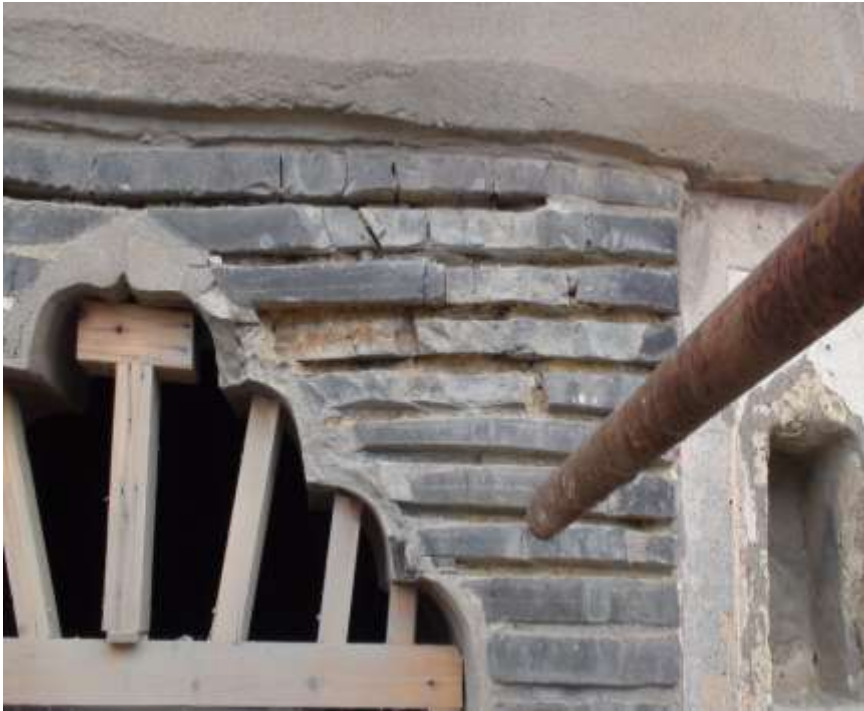
Seven grooves cut along the masonry joints
