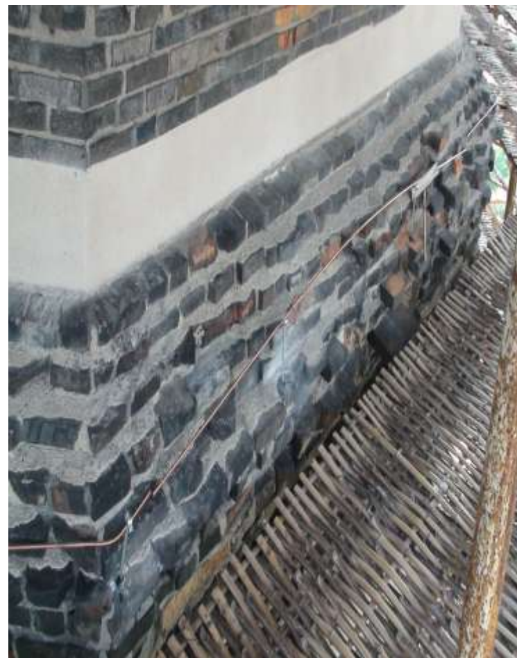
Installation of a circumferential lightning-protection band at the sixth-level eave-brick zone
