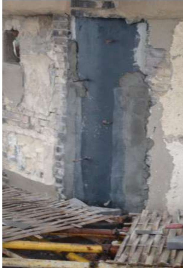
Steel wire mesh installed on both sides of the steel plate
