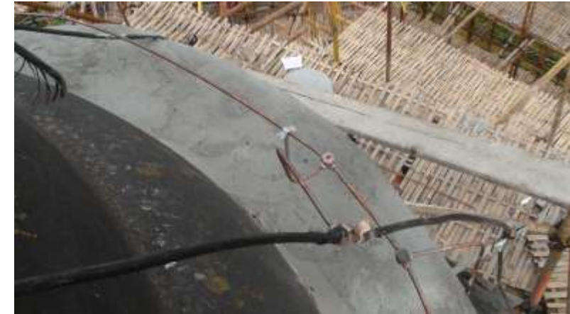
Reinstatement of the protective surface layer on the inverted-bowl element
