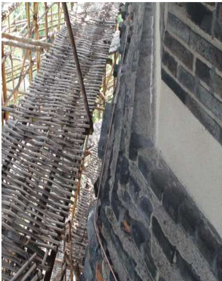
Installation of a circumferential lightning-protection band at the fifth-level eave-brick zone
