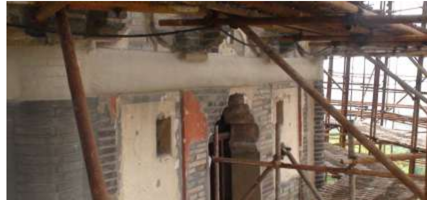
After local repair
