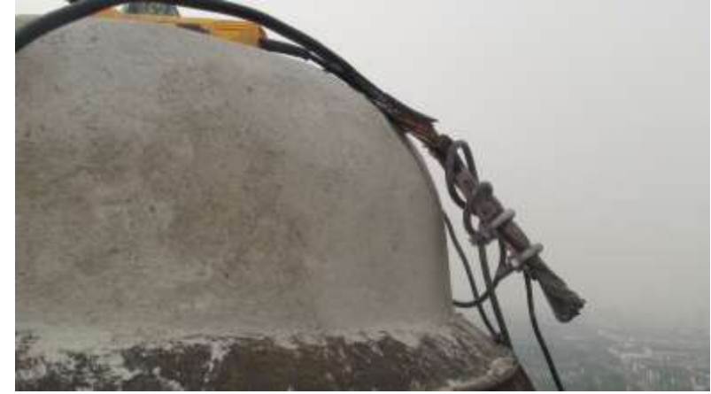
Detached and cracked areas were repaired using crack-resistant and water-resistant repair mortar.
