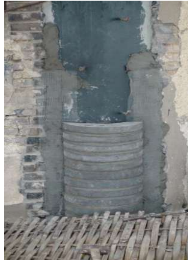
Rebuilding of a corner masonry column containing a mildly corroded steel plate
