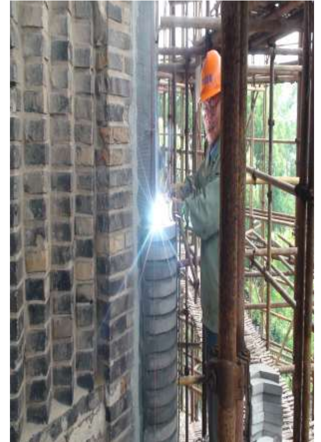
Two tie bars welded at approximately 500 mm vertical intervals
