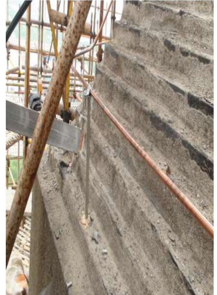
Installation of a circumferential lightning-protection band at the seventh level
