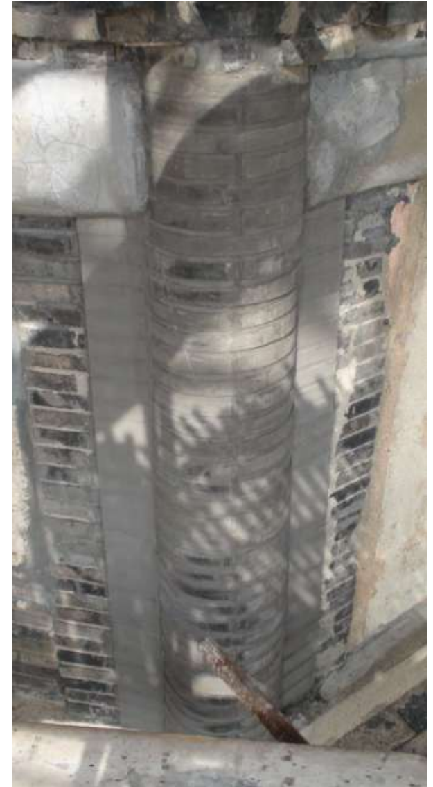
Rebuilt corner masonry column No. 5 at the fourth level
