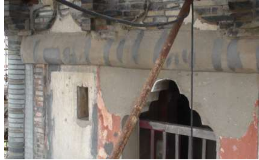
Crack repair around the circumferential steel hoop
