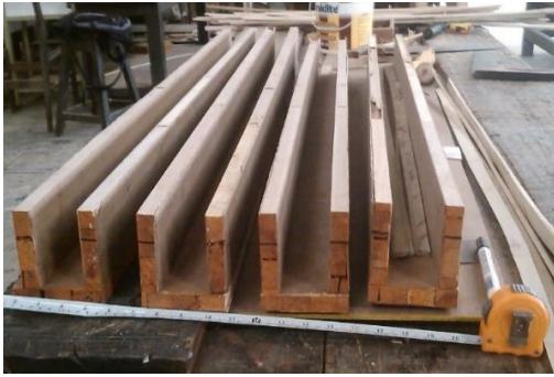
Figure 2: Custom plywood formwork designed for specimen fabrication.
