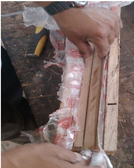
Figure 3: Layer-by-layer adhesive application and lay-up within the formwork.
