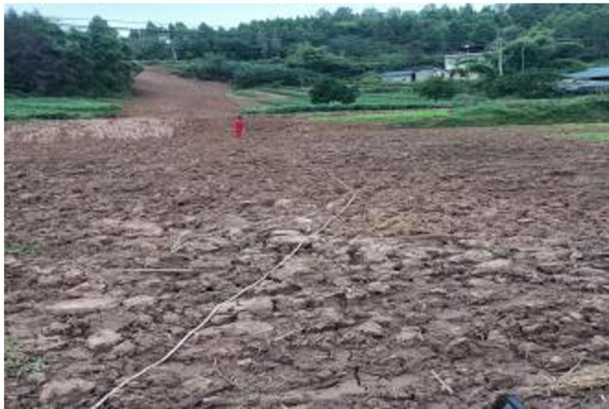
(a) Pipeline No.1
