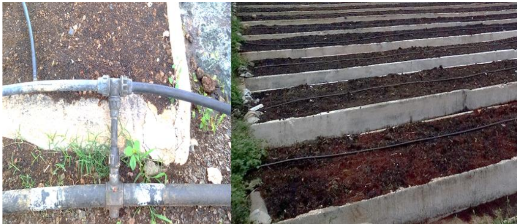
Fig. 3 Distribution pipe and laterals at the 14 July organoponic farm
