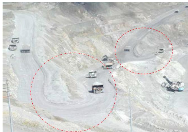
Fig. 7. Road sections with turning radii below the recommended design value along the haul routes.
