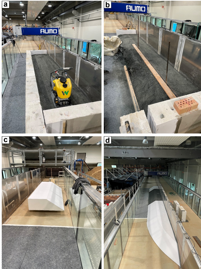
Figure S8: Experiment preparation in the high-performance morphological flume. a Compaction of the foundation body in layers. b Profiling of the foundation slope. c, d Placement of the hollow bodies.
