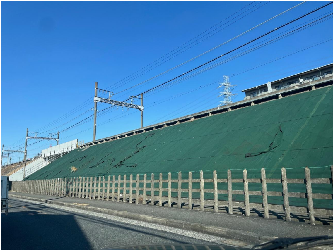
Fig. 6 Slope surface covered ground sheet, 2025 (photographed by the author).
