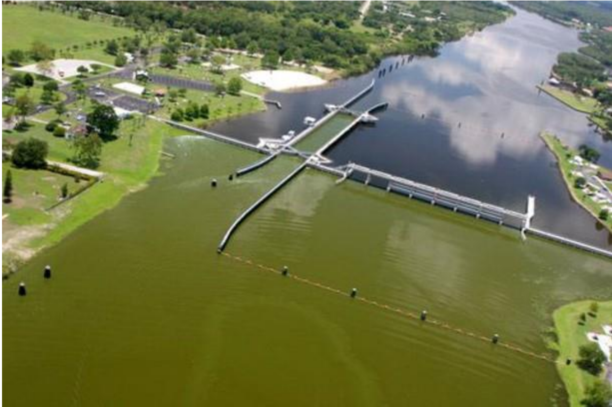
Fig. 1. S-79 water control structure in the C-43 Canal at the upper boundary of the Caloosahatchee Estuary. Bloom of the toxic cyanobacterium Microcystis aeruginosa is shown accumulating at the structure (Milbrandt, Sanibel Captiva Conservation Foundation).
