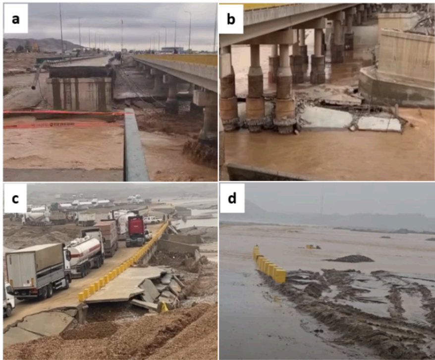
Figure 3 Damage to infrastructure (10/12/2025), a and b) Damage to the Tuz Khurmatu bridge, c) Accumulated trucks on a damaged road near the Daqooq town, and d) Inundated main road between Baghdad and Kirkuk city.
