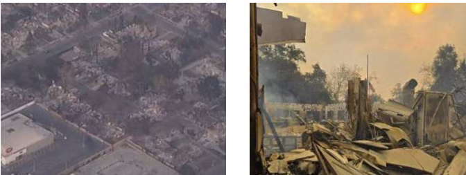
Photos 10 and 11 document extensive structural destruction within developed residential areas affected by the Eaton Fire. The observed damage illustrates the potential for community-scale fire propagation where structures, vegetation, and other combustible materials are closely interconnected within the WUI environment.
