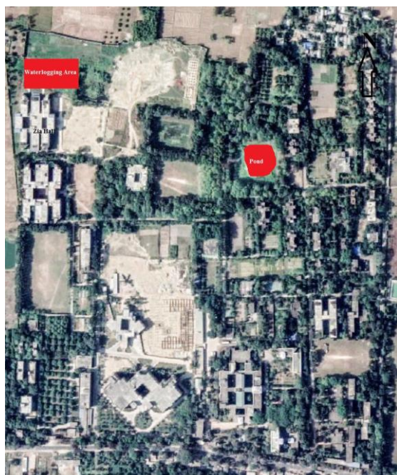
Figure 2: Aerial map showing HSTU campus and its wastewater discharge sites as red spot.
