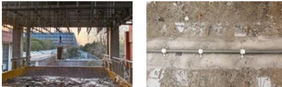
Figure 3. Rainfall and groundwater equipment.
