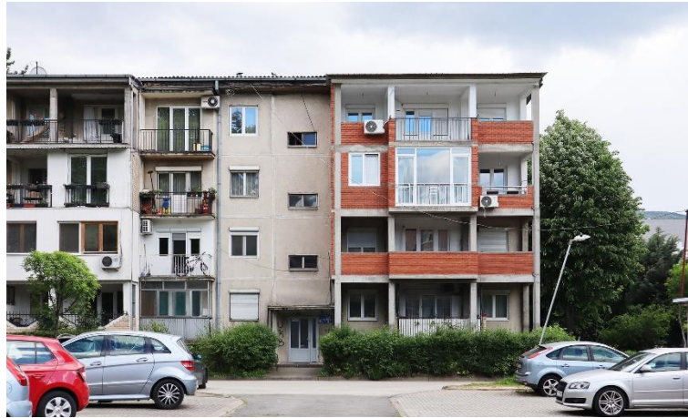
Fig. 7 Building showing a type 2 extension configuration in Karpos III: the addition of an independent structure solely at the level of the existing balconies. Photo by the author.
