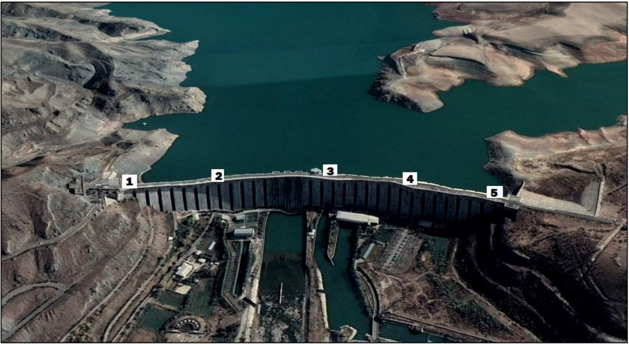
Figure 3. Microseismic measurement points at the Andijan Reservoir dam
